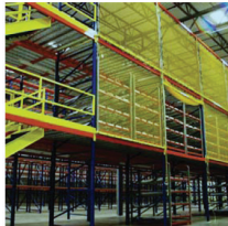
Preventing injuries from falling merchandise using designs in rack-guard netting (11)
