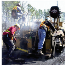
Preventing exposures to asphalt fumes with emission controls (6)
