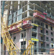
Preventing falls and fatalities with tie-in scaffolding (5)
